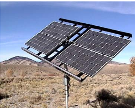
Incessantly subjected to extreme temperatures, this system provides power for a water pumping system in the US desert.
