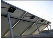
The AC PV Module is a module that combines the PV module and the micro inverter during the manufacturing process. In traditional micro inverter applications, the micro inverter is attached to the junction box on the back of the panel. With this solution, the micro inverter replaces the junction box on the PV module completely. This means you have all the advantages of micro inverters, and none of the disadvantages.
